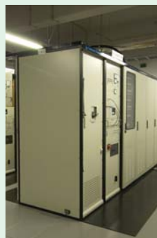
Left/ Transmitter room: Two 50-kW transmitters for operation and backup use; in the event of malfunction, the system will automatically switch to the backup unit. Right/ Time signal management block: Series of measurement machine racks for generating frequency signals and the time code for radio clocks and time comparison using the standard signal of a cesium atomic clock
