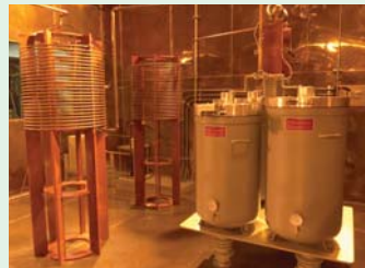
Left/ Large coil and condenser for impedance matching Right/ Converter room: The final block, which feeds the 50-kW transmission power from the converter room to the antenna. The doughnut-shaped metal structures forming a dumpling shape installed to the system act as a lightning arrester.
