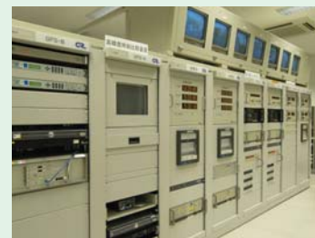
Left/ Transmitter room: Two 50-kW transmitters for operation and backup use; in the event of malfunction, the system will automatically switch to the backup unit. Right/ Time signal management block: Series of measurement machine racks for generating frequency signals and the time code for radio clocks and time comparison using the standard signal of a cesium atomic clock
