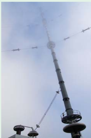
Top: Entrance gate to the facilities of the Hagane-yama Standard Time and Frequency Radio Station; the pillar on the left is the base of the 200-m antenna. Bottom: Low-frequency, standard time and frequency signal transmission 200-m antenna atop the 900-meter-high Hagane-yama summit; the top of the antenna is hidden in the clouds.
