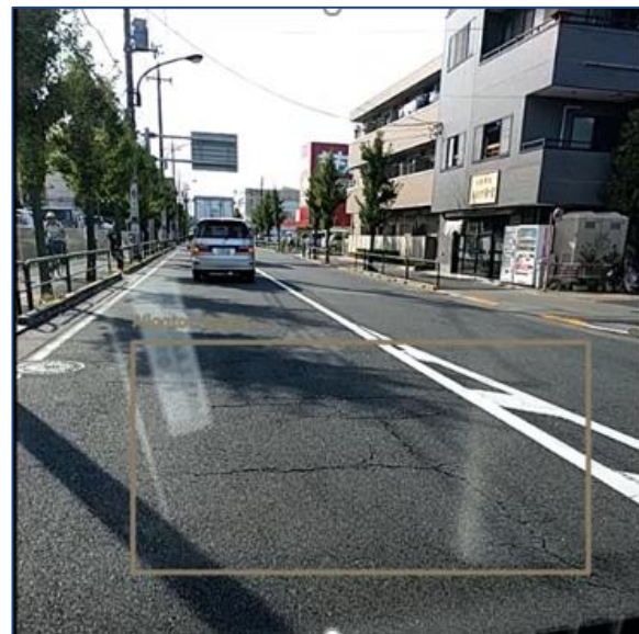
Alligator Cracks
