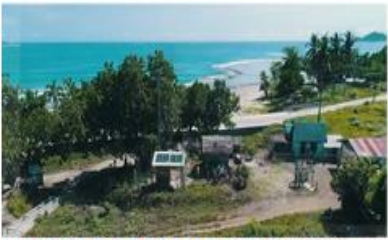
Providing communications services in last-mile areas We have provided cellular coverage to one of the most remote areas of the Philippines where incumbent telecoms are unable to profitably serve
