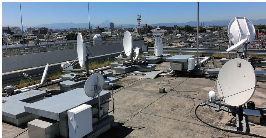
Figure 6 Two-way satellite antenna group for comparing time and frequency (Roof of Building 2, NICT headquarters)
