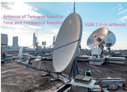
Figure2 Antennas at the roof of 2 nd building of NICT Headquarters (Koganei)
