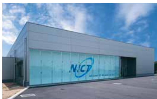
Kobe Clean Room
