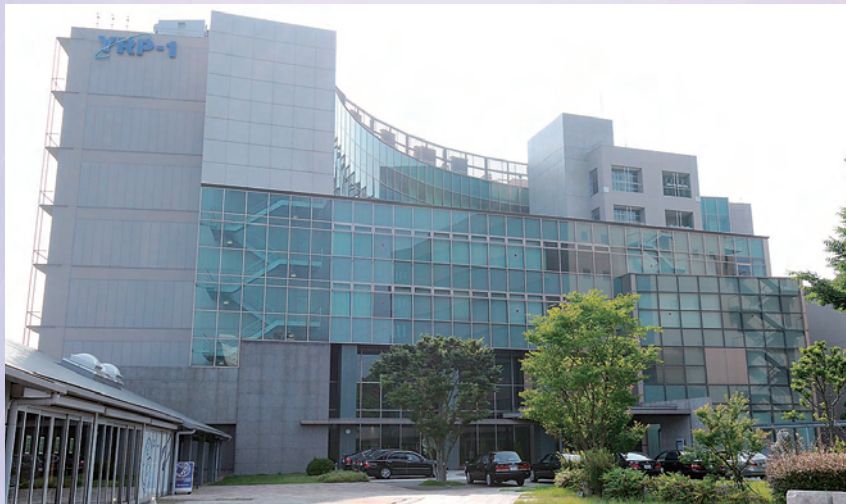
● YRP Building 1, housing the New Generation Wireless Communications Research Center
