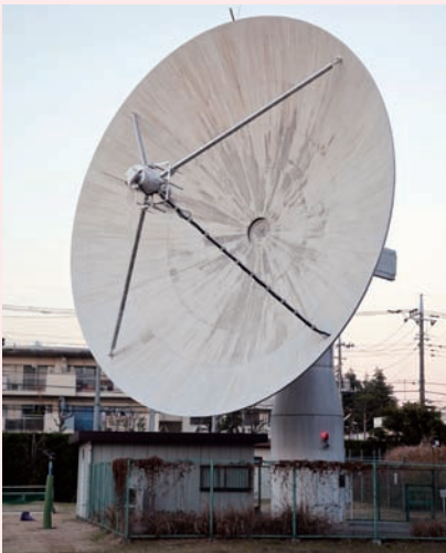
Figure 5 ● In the NICT headquarters, a parabolic antenna is installed to receive real-time solar wind data from the ACE spacecraft.
