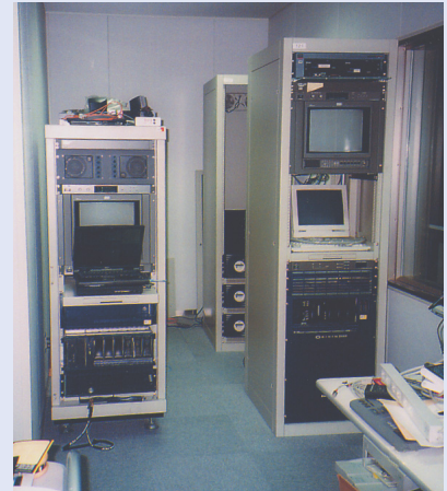
External view of Ruff Systems
