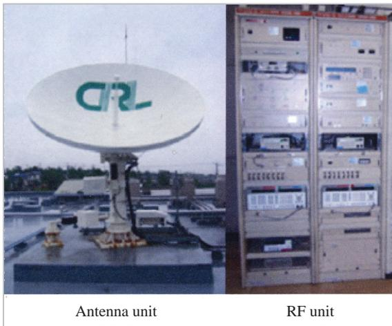
**Fig.2** Appearance of S-band earth station
