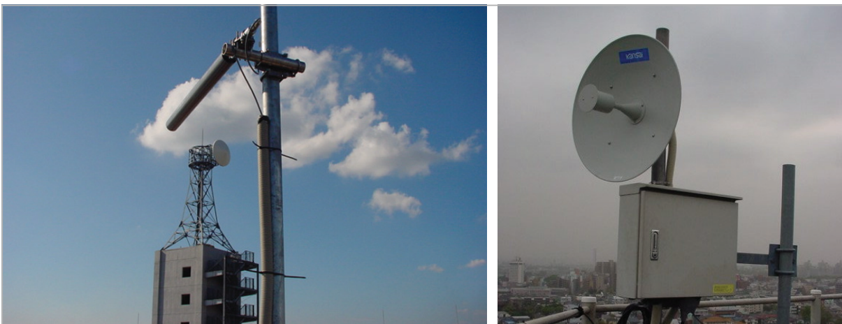
Fig.2 Long-distance wireless LAN antennas installed at NRIFD (left) and NICT (right)
