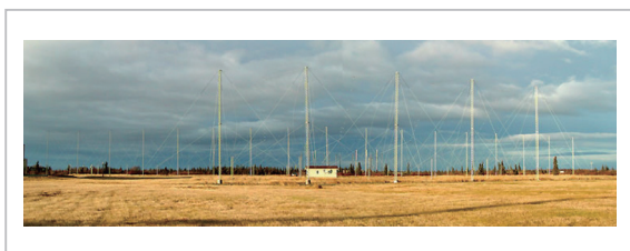
Fig.6 Picture of the radar site
