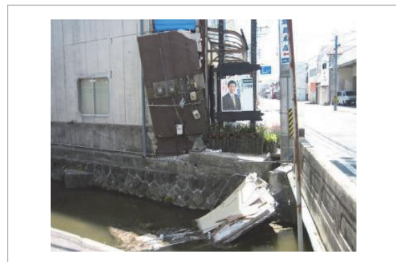
Fig.65 On-site investigation of the Iwate-Miyagi Nairiku Earthquake in 2008
