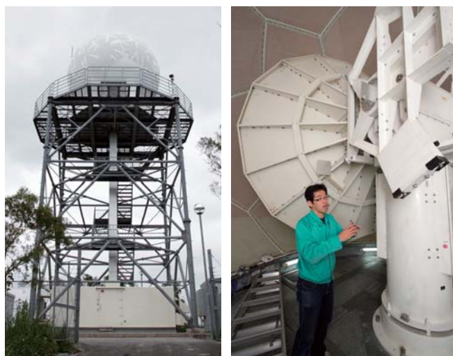
Figure 3 ● Rain radar's radome (left) and the radar (right) inside the radome.
