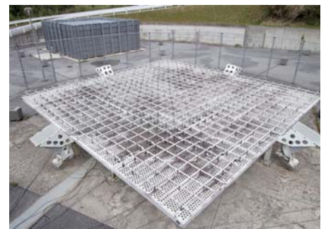
Figure 5 ● The wind profiler is installed in a valley to minimize interference from other radio stations.
