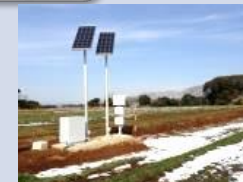
Wi-SUN Research and Demonstration Platform
