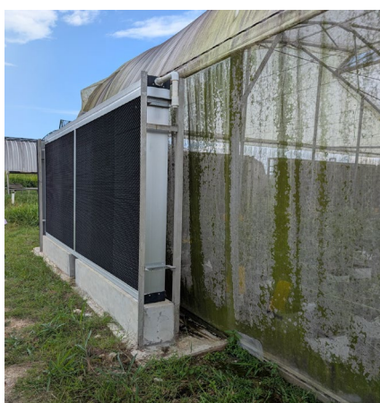
Figure 1a – Inspecting the waterwall installation.
