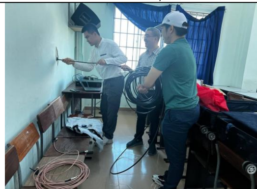
Fig. 8. GNSS cable installation inside the room (Dr. Lin, Dr. Budtho, Dr. Sophan).
