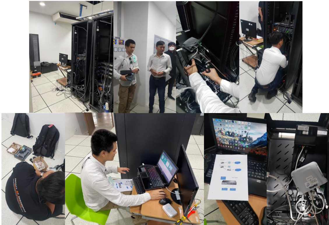
Fig. 6. Installing the new router and configuring the network connection between CADT station and KMITL's main data server.
