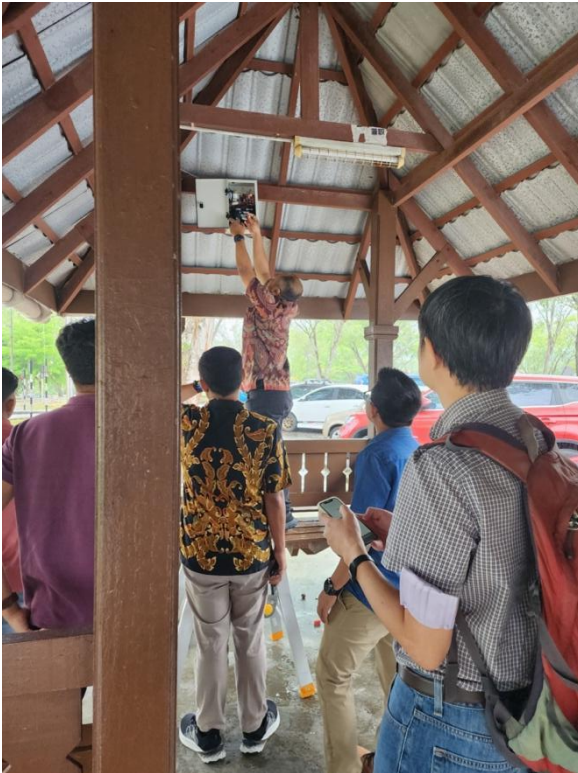
Figure 7: Inspecting the battery charging system
