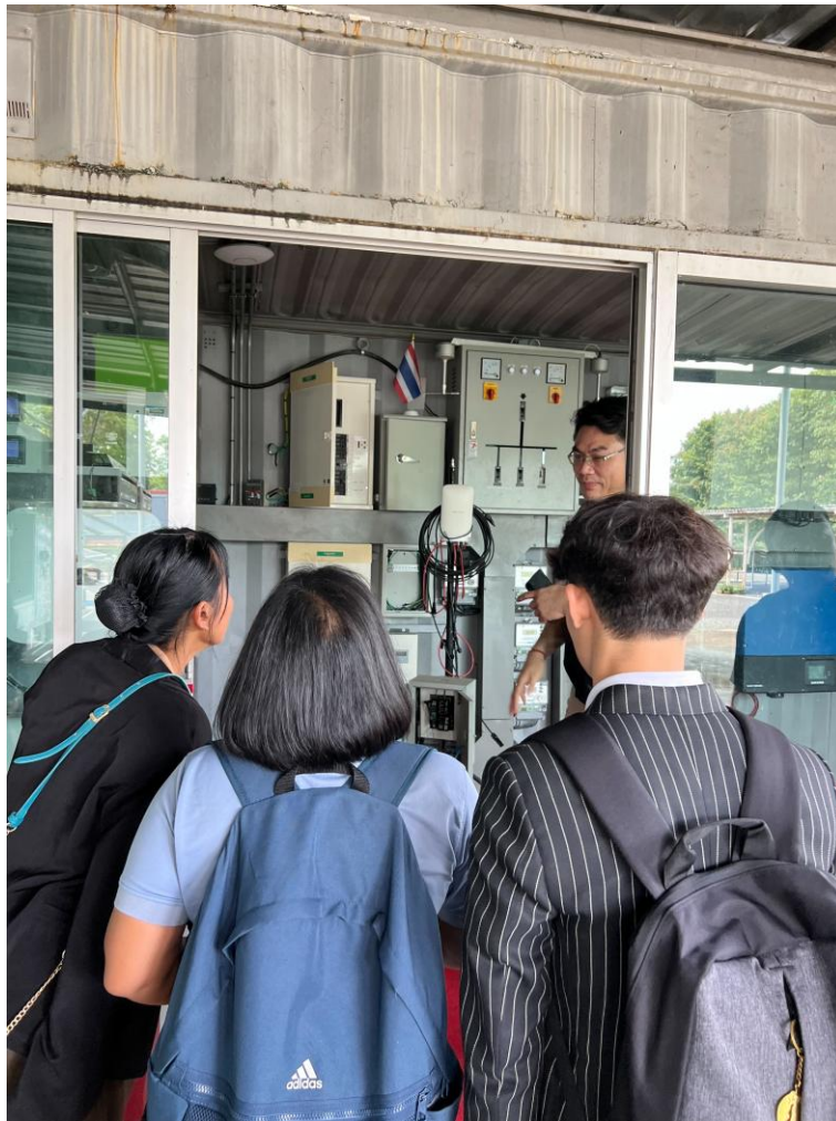
Site visit to RMUTL's Doi Saket Campus
