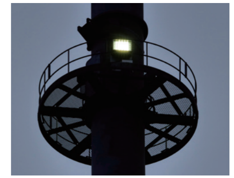
Figure 4 Aircraft warning light test (Ohtakadoya-yama Transmission Station)
