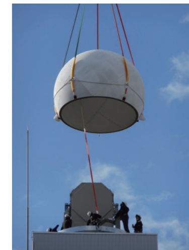
Figure 4 Installation of MP-PAWR antenna (December 12, 2022)
