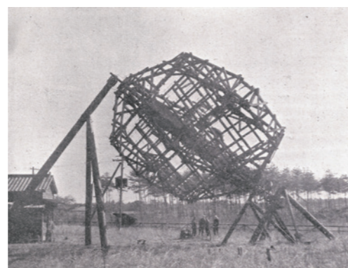
Figure 2 The Solar Noise Observation Antenna at the Electrical Communication Laboratory's Ooi Radiowave Observatory[2].
