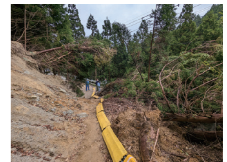
Figure 6 Landslide at Hagane-yama Transmission Station caused by typhoon
