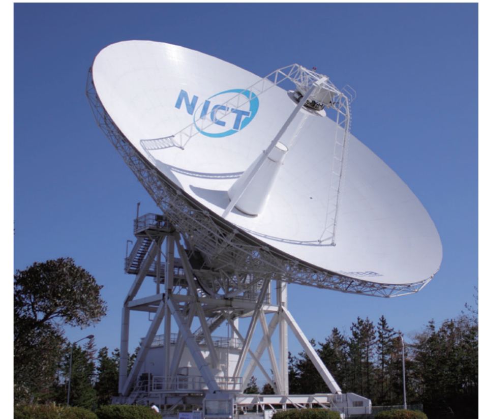
Figure 2 The Kashima 34m antenna, which has been at the forefront of the world for many years in VLBI research and development and observations
