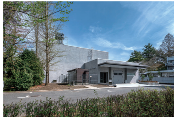
Exterior of B5G electromagnetic wave anechoic chamber facility
