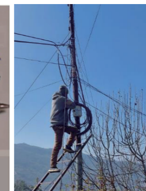
Figure 3 ITU-T L.110 environmentally resistant optical fiber cable (Left), and installation work (Right)
