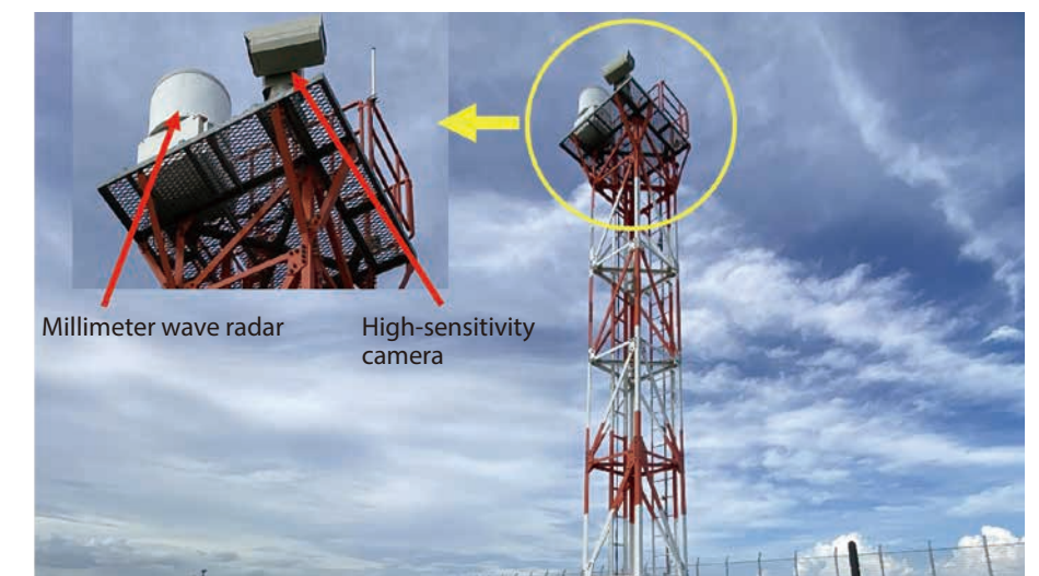
Figure Demonstration testing of a 90 GHz band radar installed at Tokyo Haneda Airport
