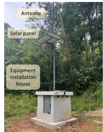
Fig.4 : An outdoor installation of one of the ten NerveNet base stations deployed in Gampola, Sri Lanka.
