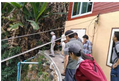
Site of Small-scale collapse
