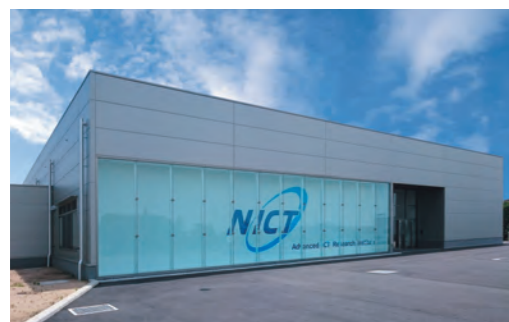
Kobe Clean Room
