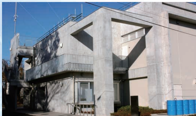
External View of Ionosphere Sounding and Trial Development Building
