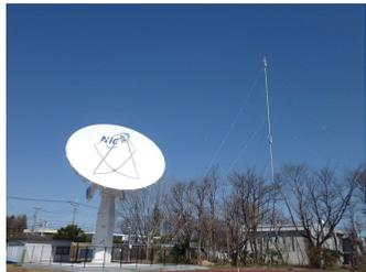
Solar wind observation satellite data receiving antenna
