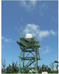
Phased array weather radar
