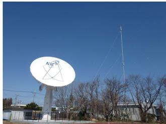
Solar wind observation satellite data receiving antenna
