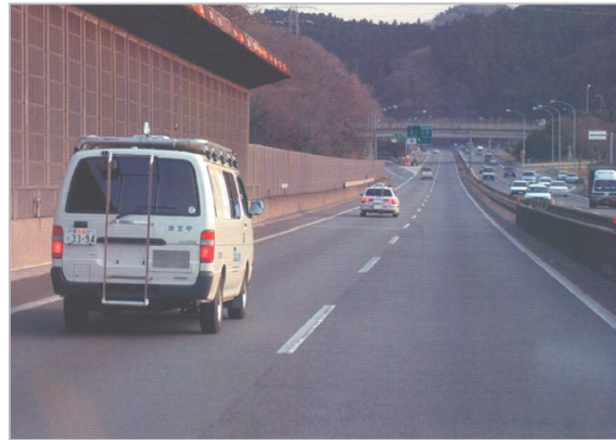
Fig. 10 View of the experimental site on an expressway
