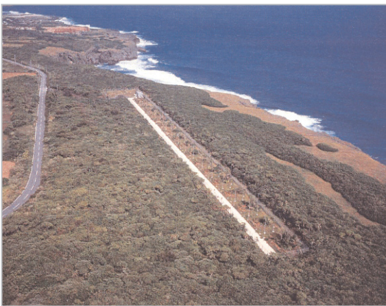
Fig.8 Yonaguni Ocean Radar Facility
