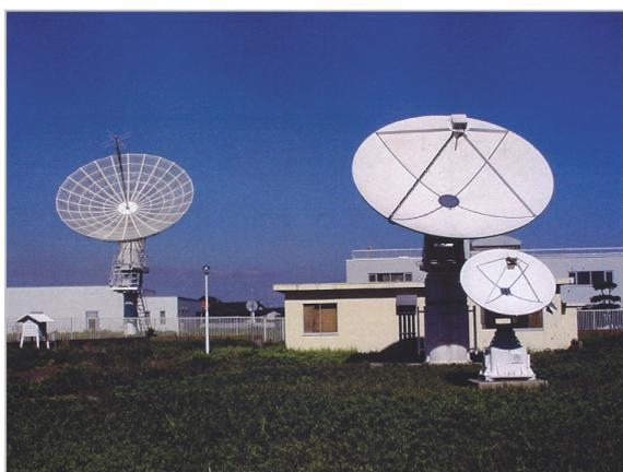
**Fig.5** The 10-m and 6-m HiRAS antennas
