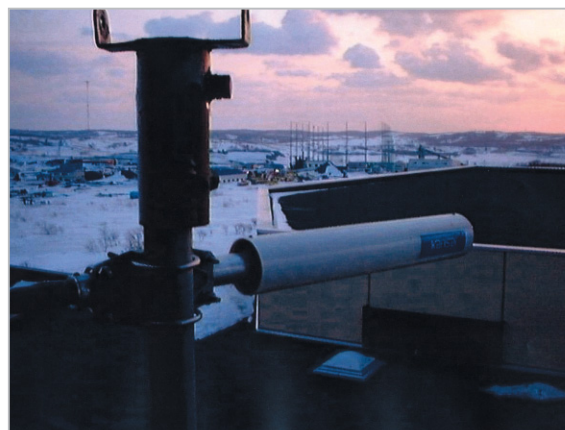
Fig.4 Yagi antenna installed outdoors for the wireless LAN to Wakkanai Otani High School (Wakkanai Hokusei)
