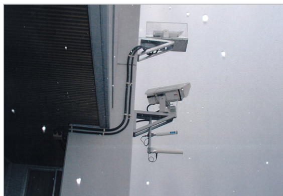
Fig.9 Duplex network equipment installed at Wakkanai High School: two sets of laser beam network equipment (for connection to Wakkanai Hokusei and Wakkanai Shoko High School) and two wireless LAN antennas for the backup link
