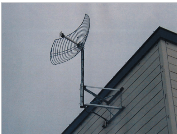
Fig. 12 Parabolic antenna installed at Soya Junior High School for long distance wireless LAN
