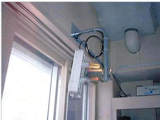
Fig.5 Planar antenna installed indoors for the wireless LAN to Wakkanai Shoko High School (Wakkanai Higashi Junior High School)
