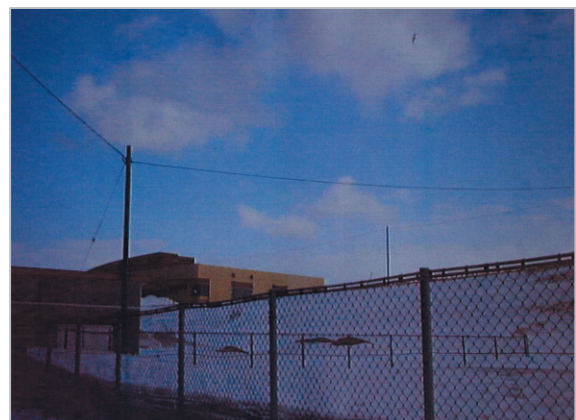
Fig.6 Fiber-optic cables connecting Wakkanai Hokusei (center) and Shiomigaoka Junior High School (to the left beyond the frame of the photograph)
