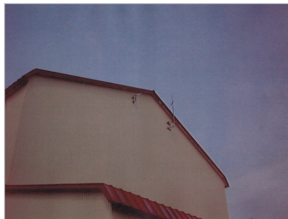
Fig.3 Relay antennas installed on the roof of the gymnasium of Wakkanai Otani High School. The antenna on the left is for connection with Wakkanai Hokusei and the antenna on the right is for connection with the Wakkanai Radio Observatory.
