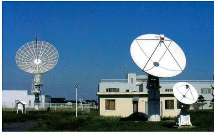
**Fig. 10** 10-m antenna (background on the left), 6-m antenna (background on the right,) and 2.8 GHz fixed frequency observation antenna (foreground on the right) of a HIRAS system
