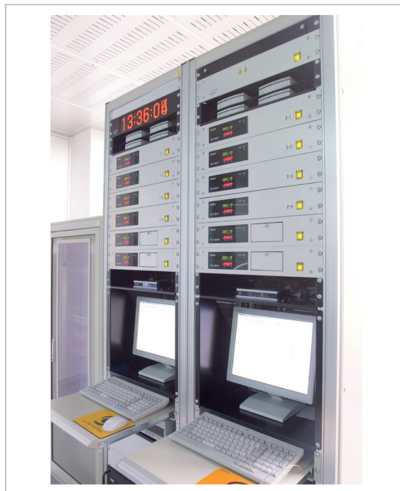
Fig. 11 Telephone JJY system
