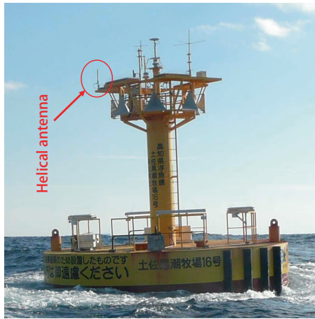
Fig. 11 Exterior of a marine buoy and the status of antenna installation
